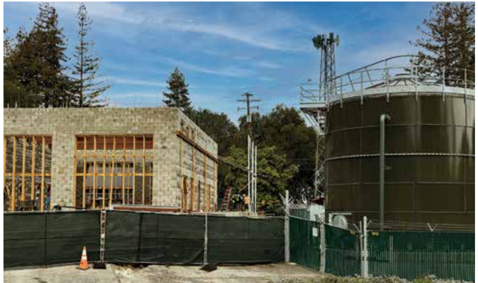
Construction of the new Redwood Estates Fire Station is moving along.
